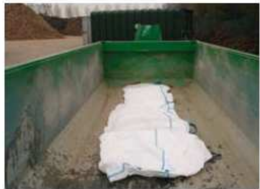
Stap 2: Containerliner in de container leggen en flappen over containerranden leggen.
