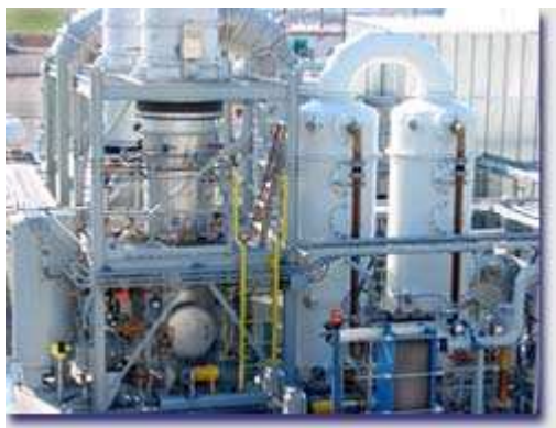
Figuur 26 Off-gas processing system (quench cooler and packed-bed scrubbers) (Bron: http://www.aritechnologies.com/tech_and_services/procassecon.htm )
